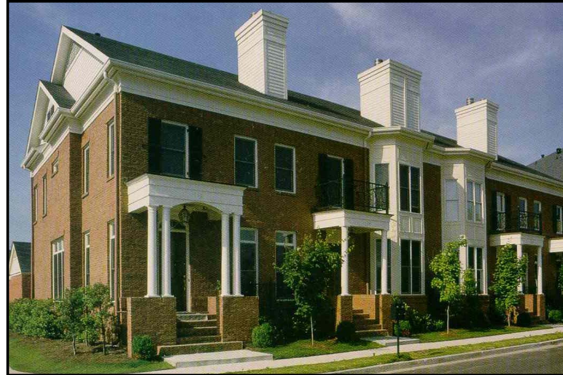
Photograph 2: These 2-story attached homes with a masonry exterior utilize wood porches and bay windows to provide variety to the building facade. (Note that the front yard setback in this photo is shallower than land use planning policy in Western Springs recommends)
