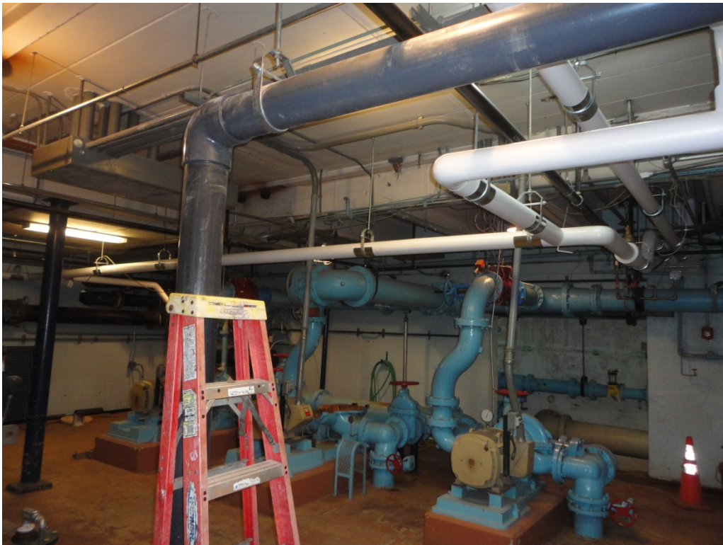
Installation of Insulation of Potable Water Lines
