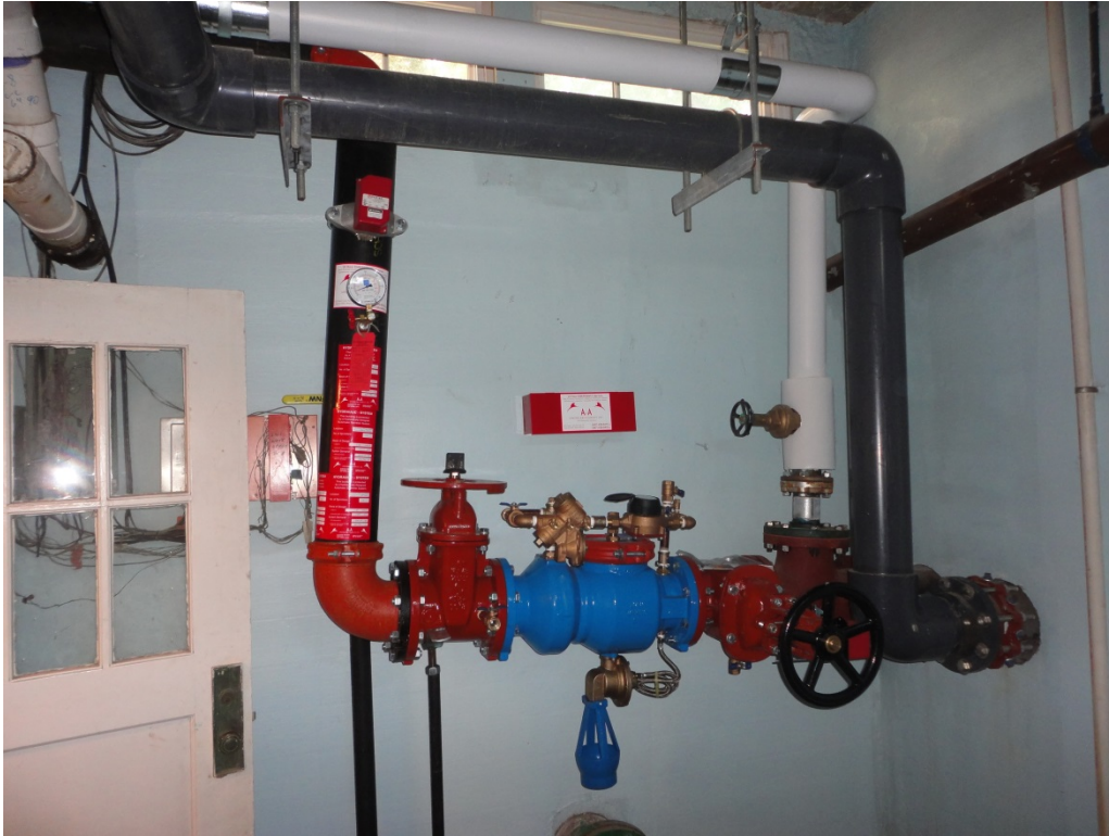
Installation of Fire Protection Backflow Preventer
