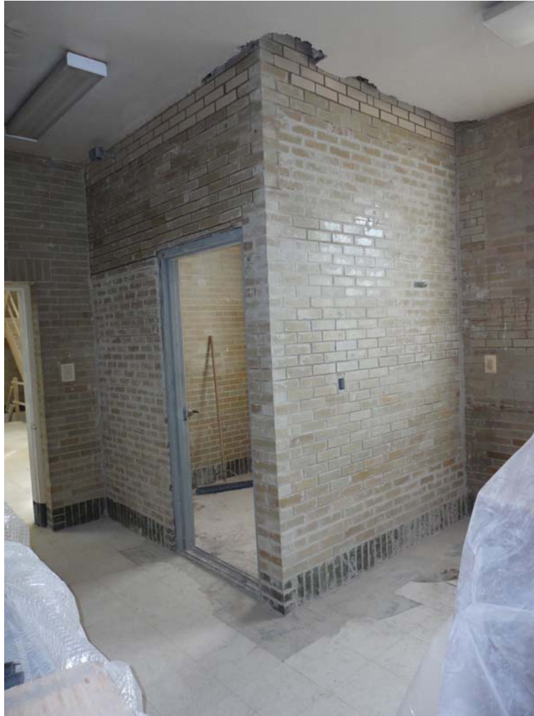
1 st Floor Bathroom Walls
