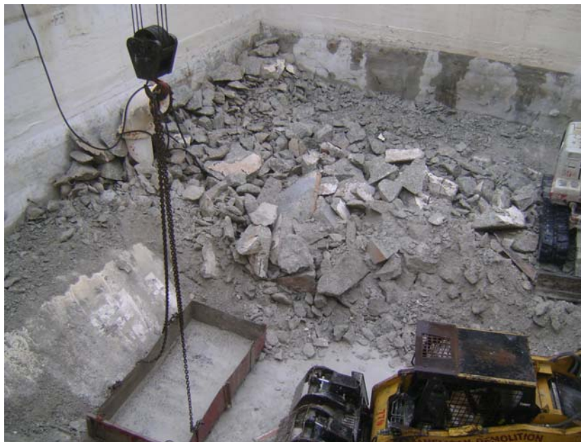
Concrete Fillet Removal
