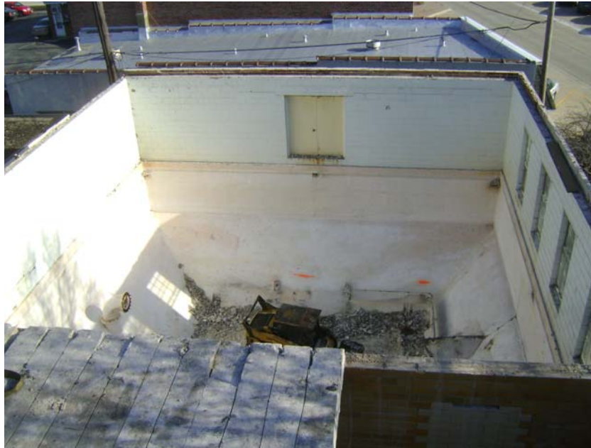
Clarifier Demolished and Removed
