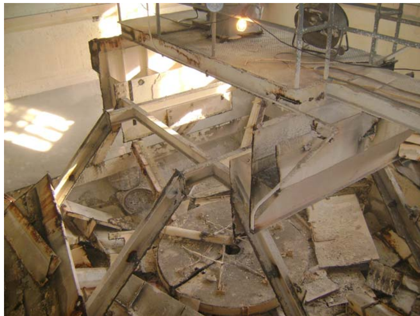
Demolition of Clarifier
