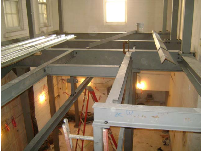
Structural Steel Installation in Raw Water Treatment
