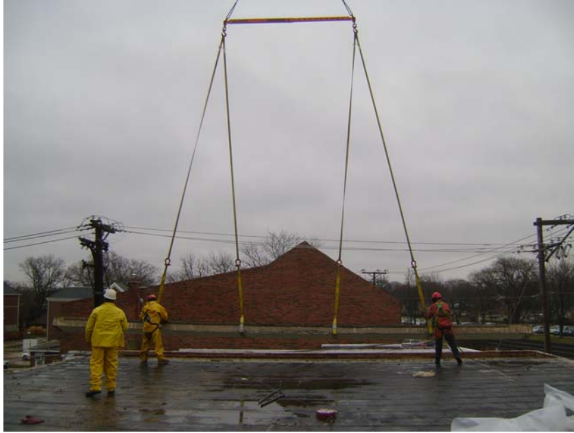
Clarifier Roof Plank Removal
